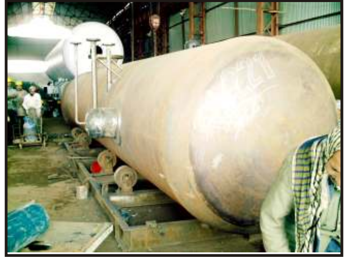
FABRICATION OF PRESSURE VESSEL
