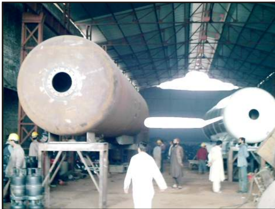
LPG BOWZER FABRICATION
