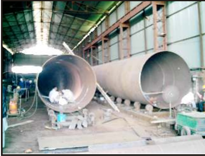
LPG BOWZER FABRICATION
